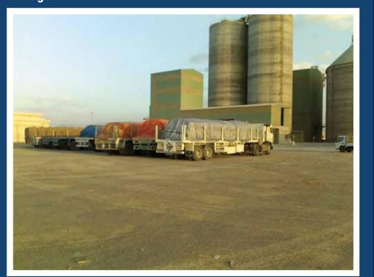
Cement Silos: Capacity of 8,000 Tones Each Clinker Silos: Capacity 30,000 Tons
